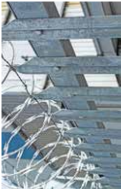
Palisade Fencing with Razor and Barbed Wires
