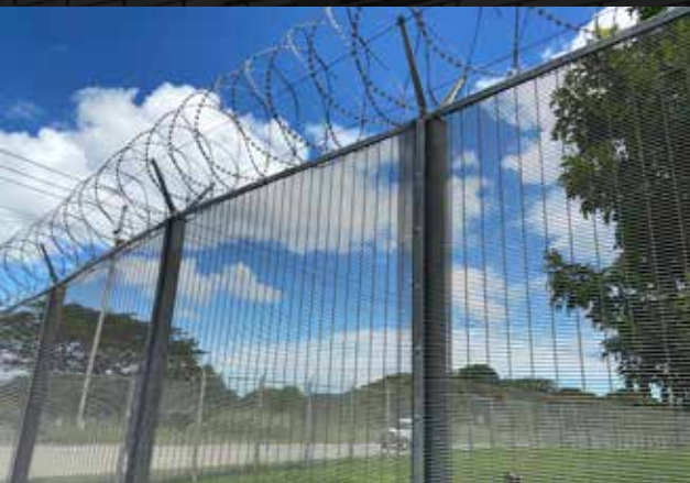
358 High Security Fencing
