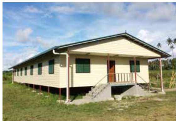
Low Set Dormitory Channel College-Kokopo, Rabaul
